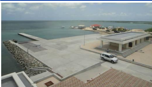
Landing Jetty and Mooring Sea Wall (Jun, 2011)
