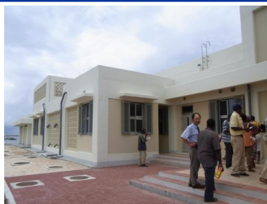
Fish Handling Building (Aug, 2011)
