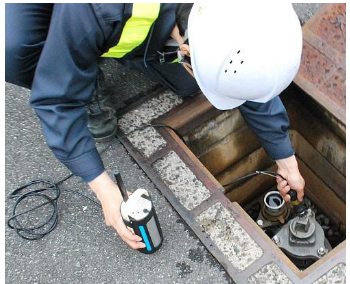
Water technician using Fuji Tecom's Pipeline Leak Detection technology.
