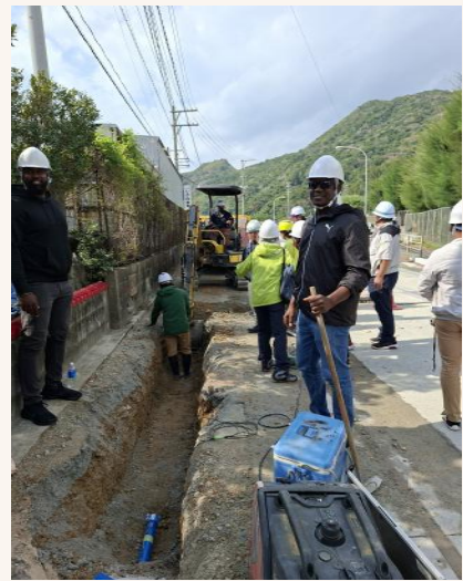
Mr. Jeffery Browne, APUA representative, engaging in a pipe laying field exercise.
